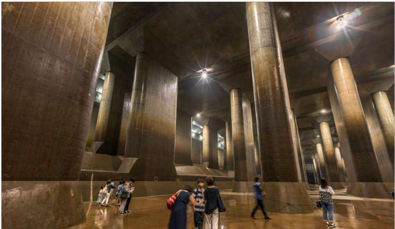
Tourists visiting the the Metropolitan Area Outer Underground Discharge Channel in Tokyo. The system has 6.3 km of tunnels and huge tanks to protect north Tokyo from flooding, Japan, 28 August 2018.
