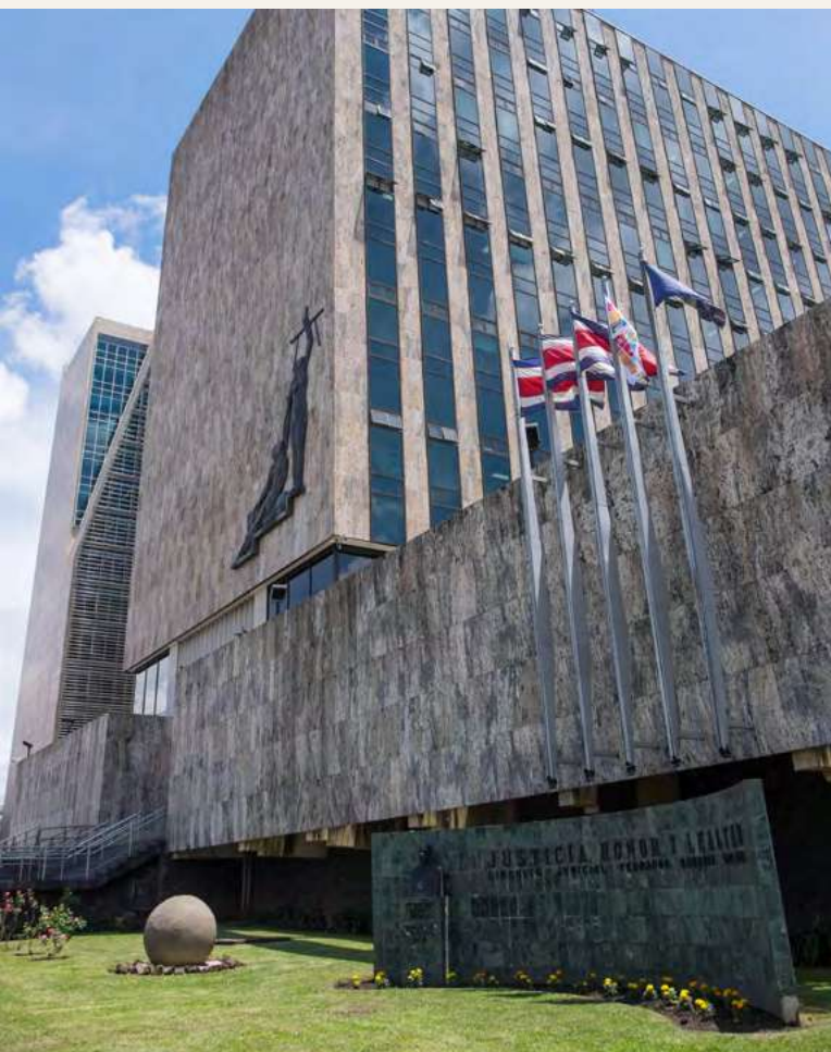
The Supreme Court of Justice building, San José, Costa Rica, September 2022.
